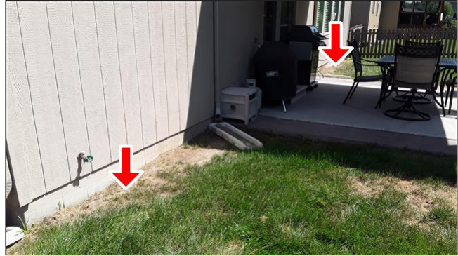
1.0 Item 2(Picture) - Landscaping is flat on West side of home
