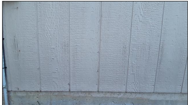
2.1 Item 2(Picture) - Close-up of exposed nails and open gaps on North side of home
