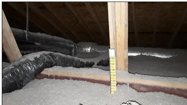
5.1 Item 1(Picture) - 13 inches of blown cellulose insulation in attic
